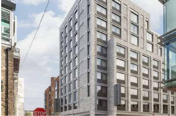
Premier Inn Gloucester Street, D2 (OPEN March 2023) Bedrooms: 113
